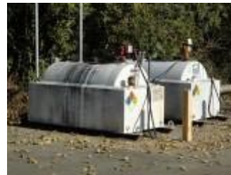
Maintenance building (fuel storage)
