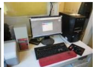
Irrigation central controller
