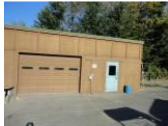
Maintenance building (pesticide storage)
