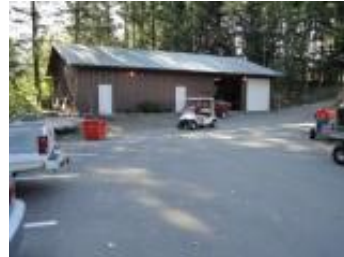
Maintenance building (storage building)
