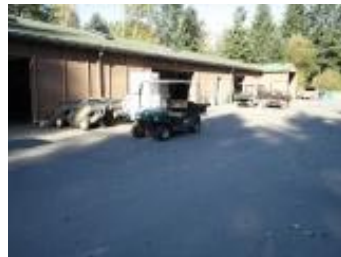
Maintenance building (Main)
