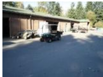
Maintenance building (Main)
